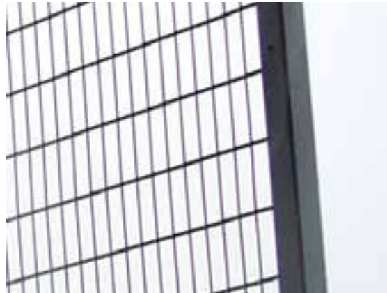
Steel construction: Hot-dip galvanised and powder coated
