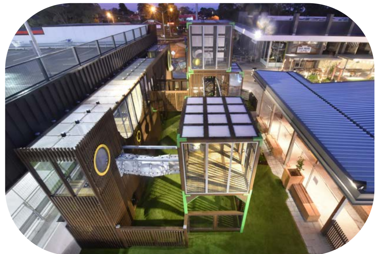
Karingal Hub – Photo by our channel partner Lark Industries, Australia.
